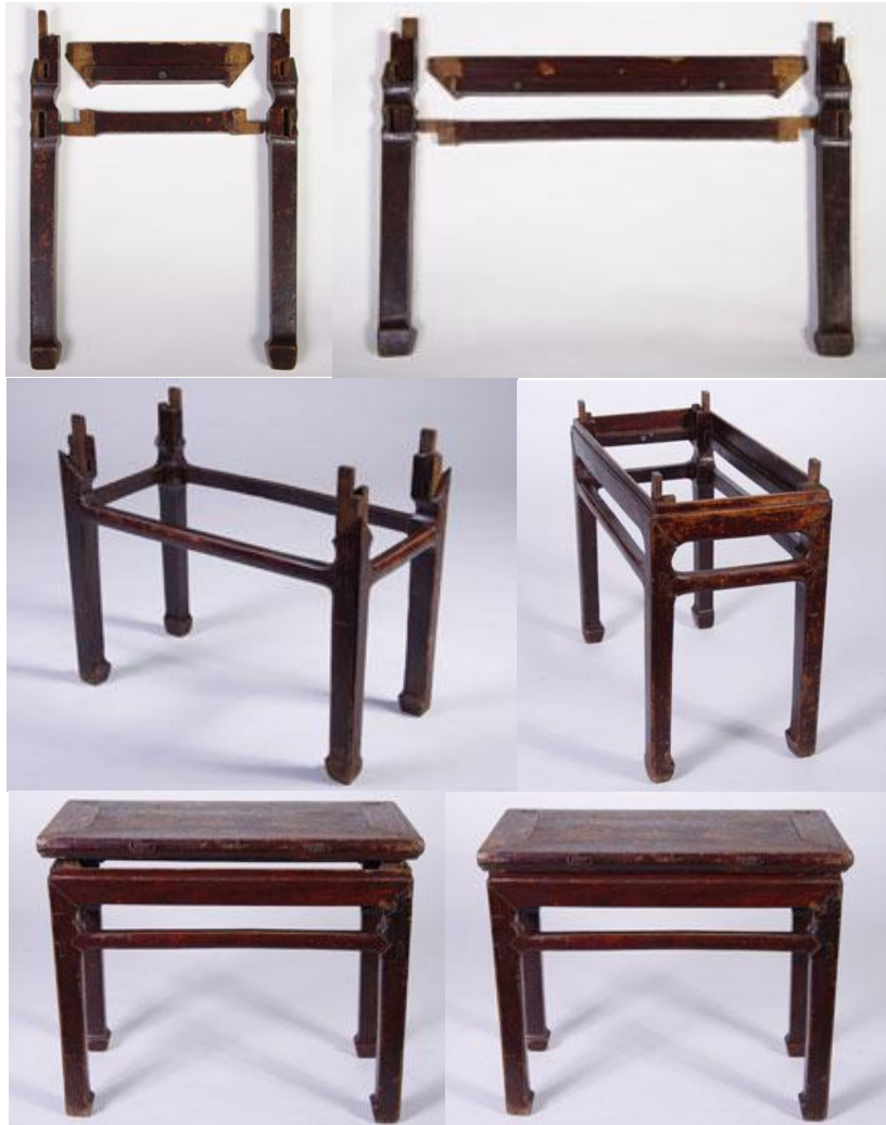
Figure 21. A stool case with a complete M & T structure.
