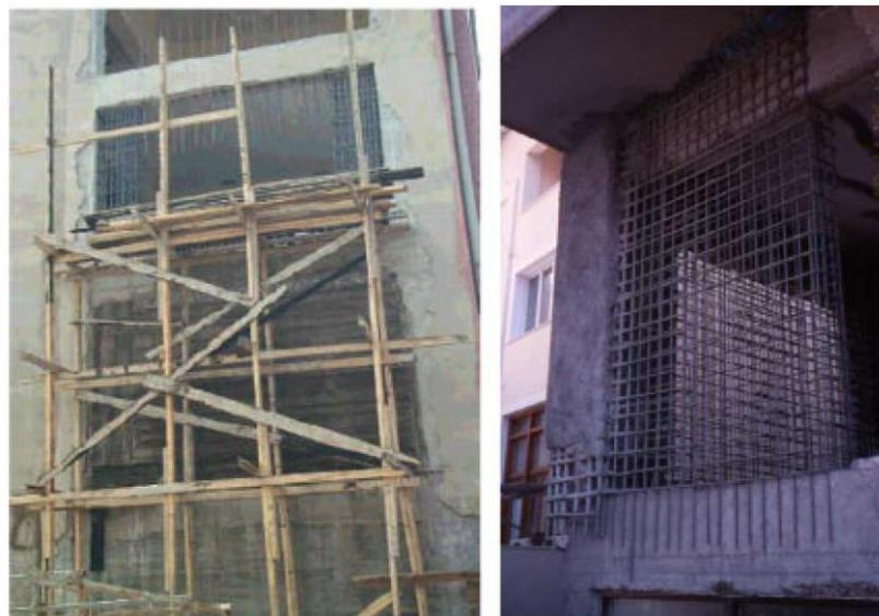
Figure 2-7 Cast in place shear wall for the retrofit of RC frames [78]
