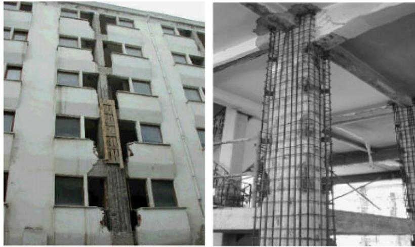
Figure 2-6 examples of Reinforced Concrete jacketing retrofit for RC frame[78]
