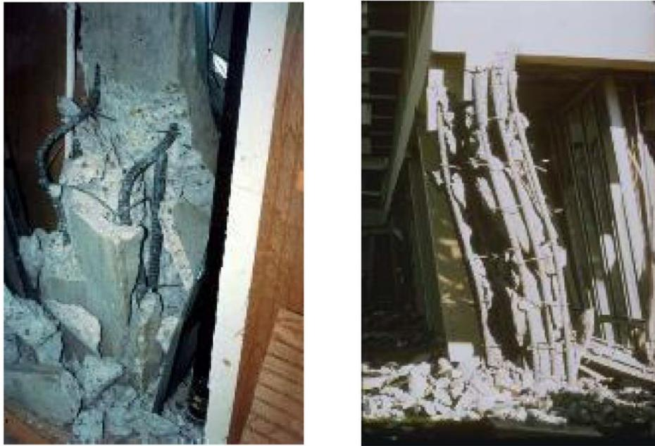
Figure 2-1 Examples of failure of poorly reinforced columns in past earthquakes[72]:
