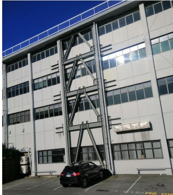
Figure 2-8 Conventional Strengthening of RC frame using EBF (Massey University Library, Wellington)
