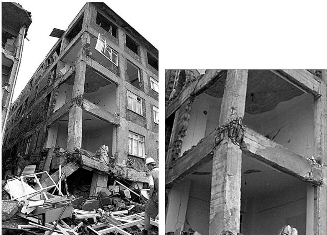
Figure 2-3 building collapse during 1999 Kocaeli earthquake in Turkey[74]
