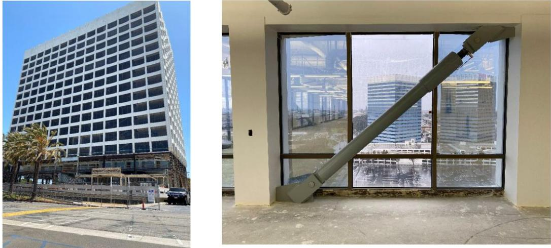
Figure 2-11 Exterior view of a 17-story building and the installed FVD[88]
