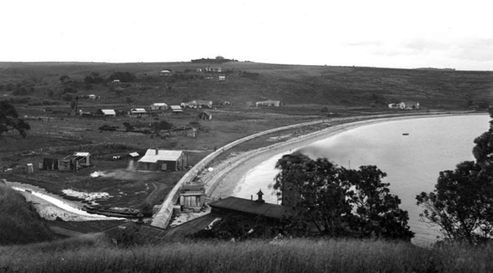
Figure 7: James D Richardson, 12 Feb 1921, Looking south west from Takapararua point across Okahu Bay showing Orakei Pa and the sewer running along the foreshore.
