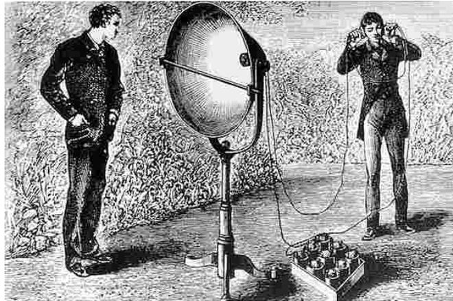
Figure 1.1: First wireless telephone conversation via photophone in 1880 [1].
