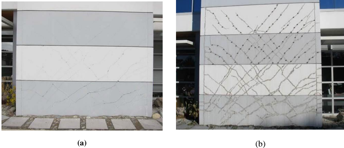
Figure 1. 6. 2011 Christchurch earthquake (a) a moderately damaged concrete shear wall [2]. (b) Crack epoxy grout injection repair for the same wall [4].
