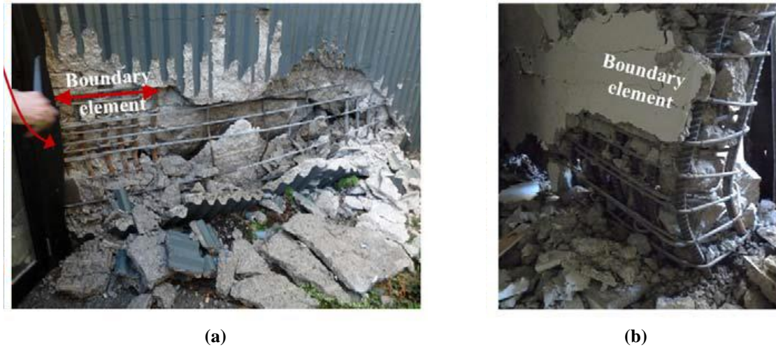
Figure 1. 3. out of plane buckling of the boundary element of a ductile designed concrete shear wall [2]. (a) damaged wall; (b) close-up of the buckled region.
