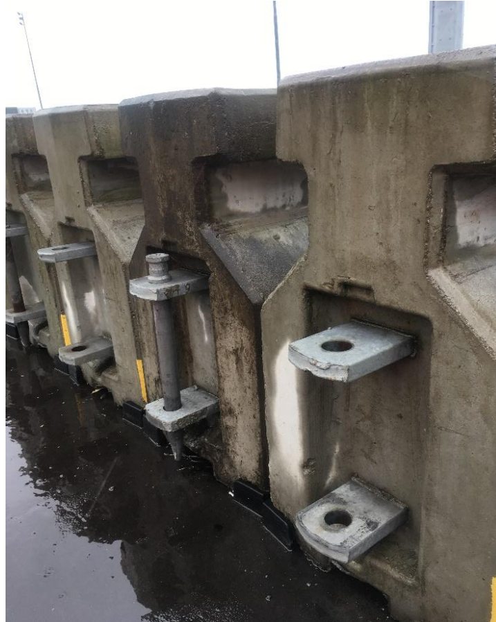
Fig. 1: Movable concrete barrier joints and metal pins.
