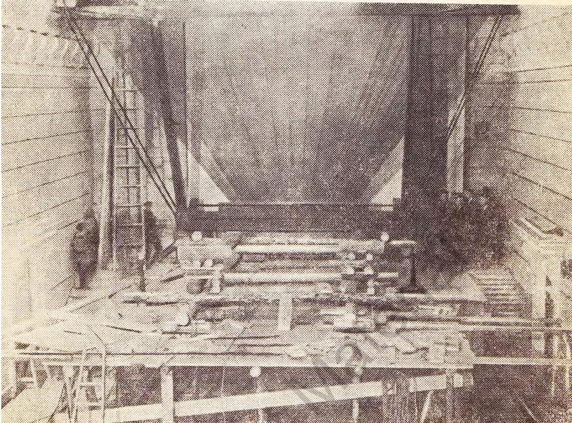
**Figure 20:** Construction of the radial raster barrier at the Moskva cinema (Moscow) *circa* 1940. The completed barrier weighed ~6 Tons. The opaque regions were formed from groups of copper wire and in total ~150 km of wire was used (Ivanov [1941]). Given the required accuracy and the lack of today's lightweight plastics the development of this barrier represents a remarkable technical achievement. (Image reproduced from Ivanov [1941].)
