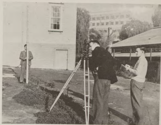
Senior Civil Engineering Students using a Theodolite and Levelling Staff
