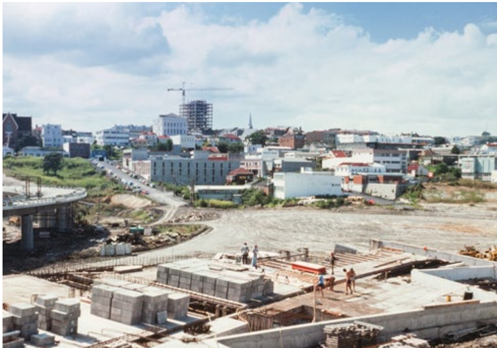
Figure 28 Looking south-east across Newton from Karangahape Road, ( Donovan, 1976). Image showing the sand belt poured for the construction of the motorway junction. Historical link roads can be seen restructured into dead ends.
