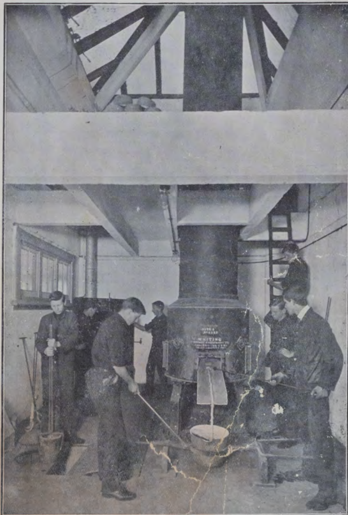
FOUNDRY PRACTICE—THE CUPOLA AND BRASS FURNACE.
