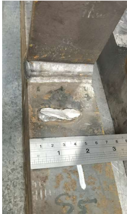
Figure 82: Unfinished steel surface with spur on the flange base plate
