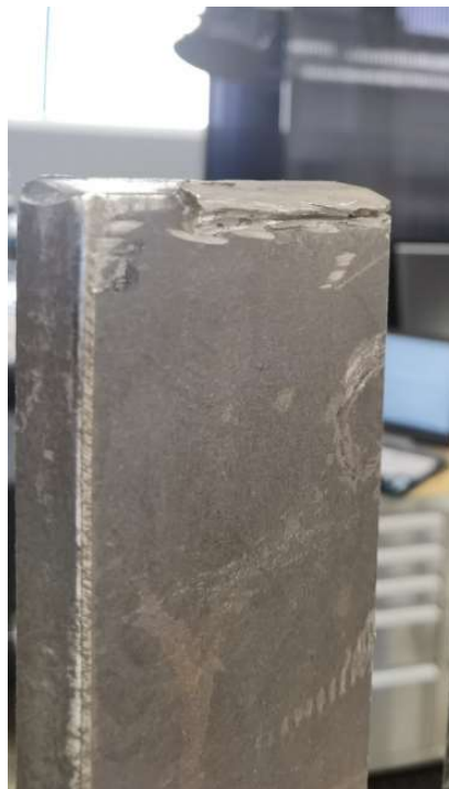
Figure 83: Unfinished steel surface with spur on the stem web plate
