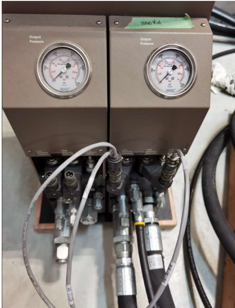
Figure 50: The pressure gauges of an HSM in AUT labs
