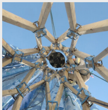
Figure 16: The structural framework of the Living Knitwork Pavilion, MIT, 2023
