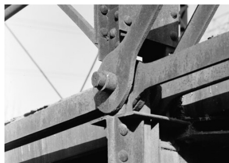
Figure 75: Hinge/ pin connection
