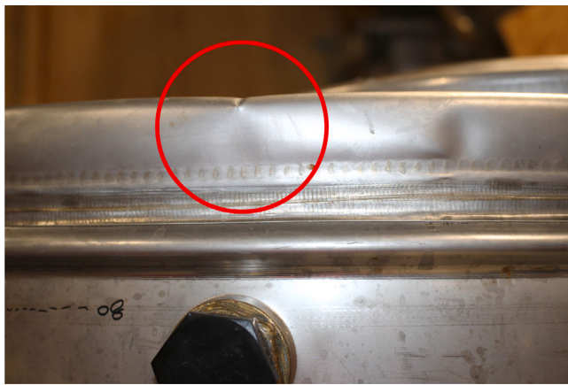
Fig. 16. Crack formation at the base plate during tests under the Christchurch 2011 0.30g.
