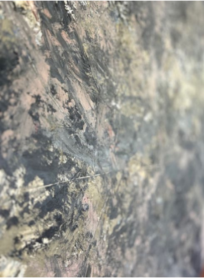
Figure 18. Detail, eventual work covered up.
