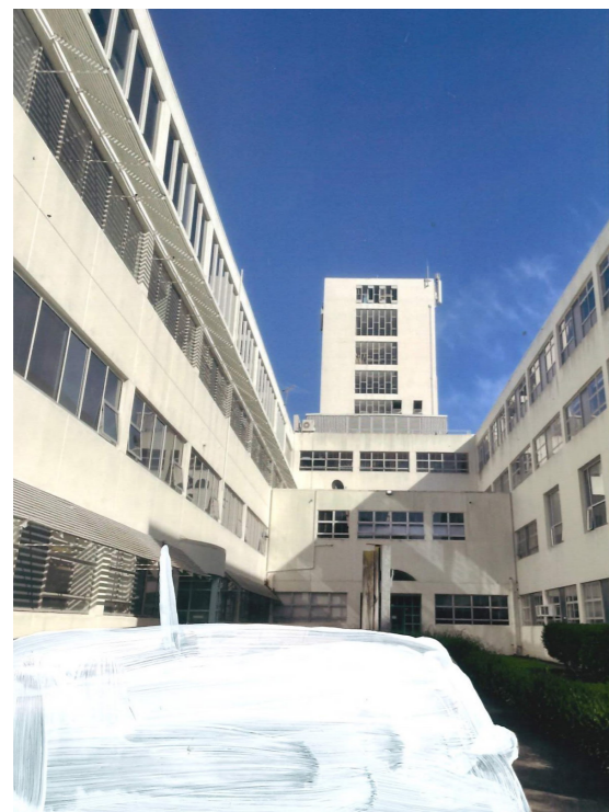
Fig. 1 Photo of Building 16 courtyard from road. Car painted over to show general volume of vehicals in line of site at human scale.
