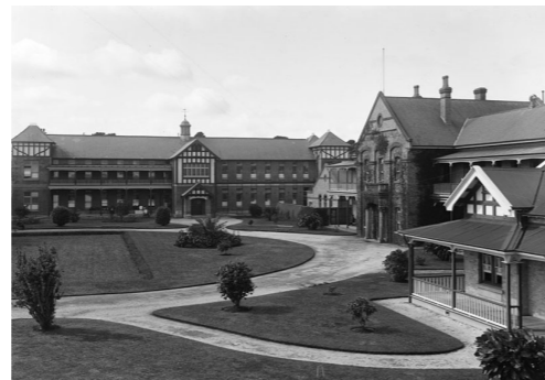
Fig. 4 Photo of Infirmiry Ward for Incurables (left) adjacent to the costley home for the aged poor (right) April 1918. 16
