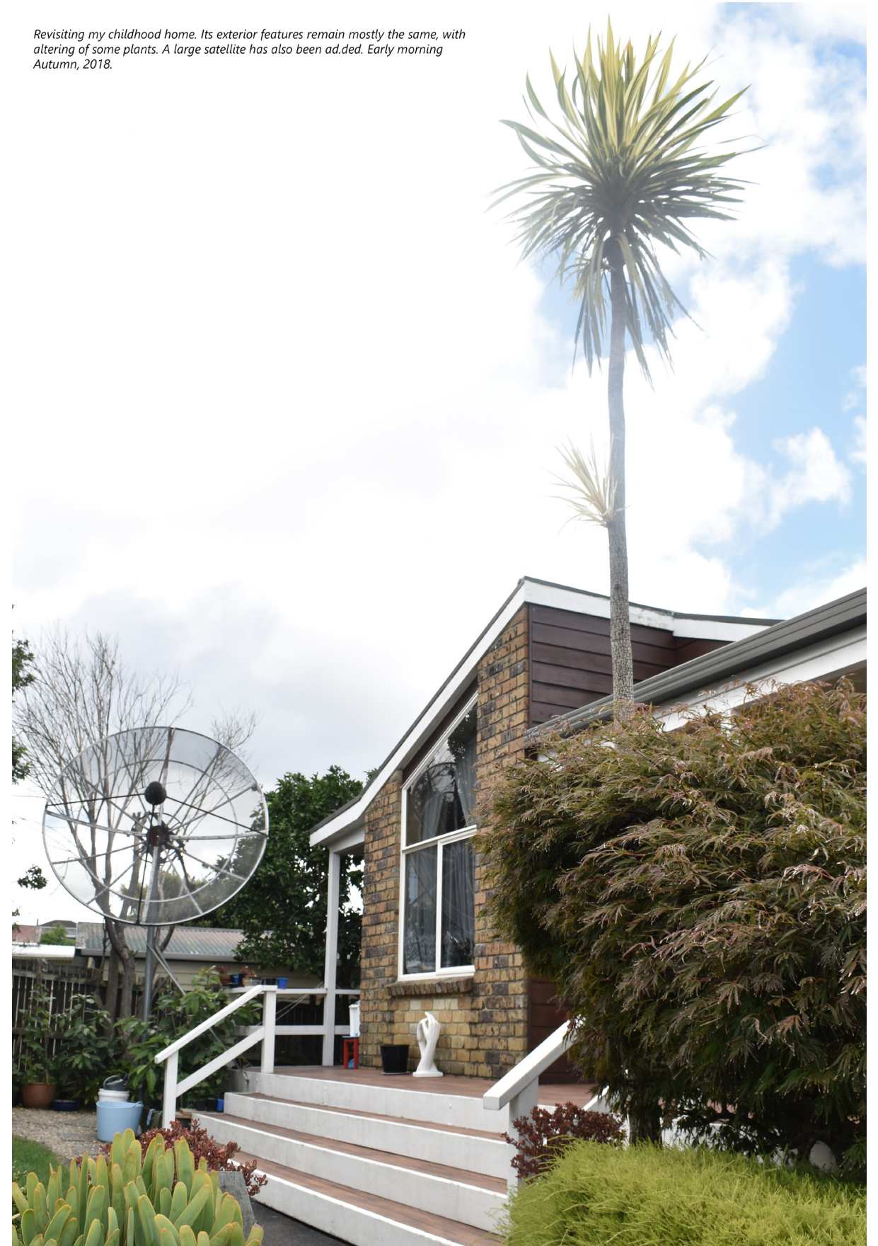
Figure 2.4: Approaching the front deck Liu, Frank. 2018
