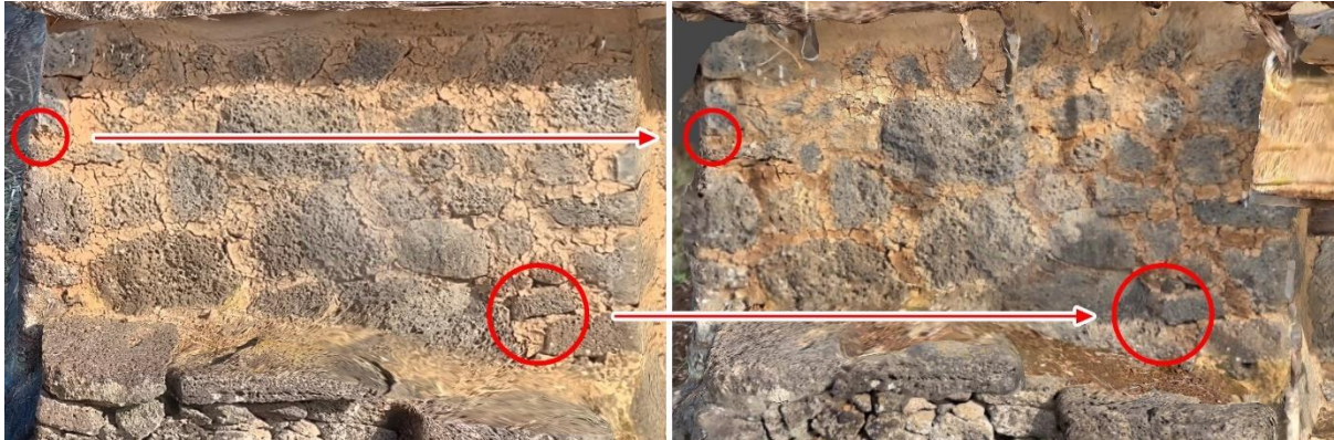
Figure 79. Compatible matching points for aligning geometry data between videogrammetry (left) and MLS (right) output
