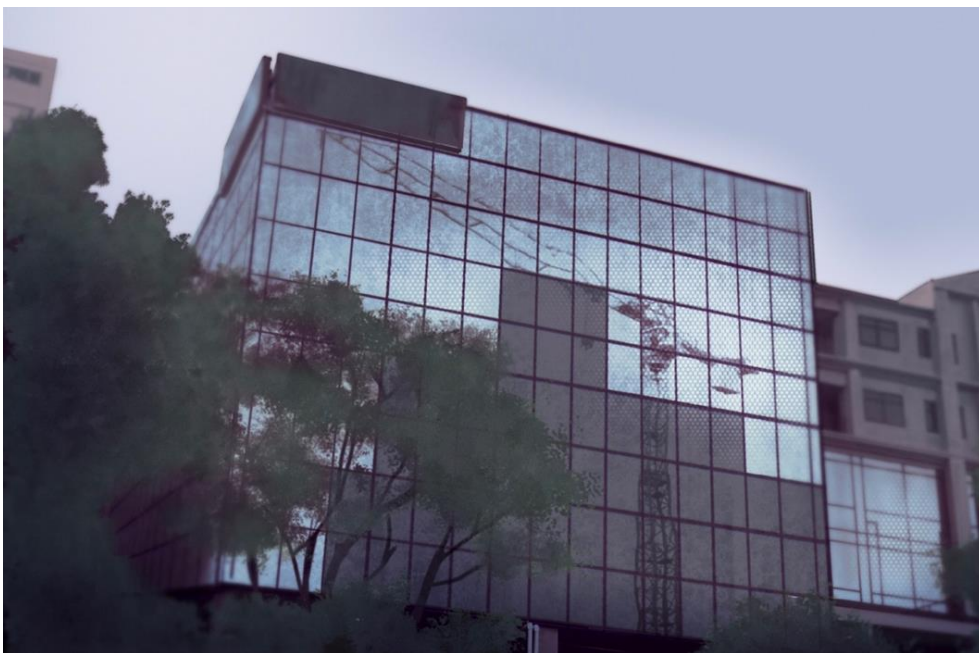
Figure 23. Bixley, O. (2022). Crane Reflection . [Digital Painting].
