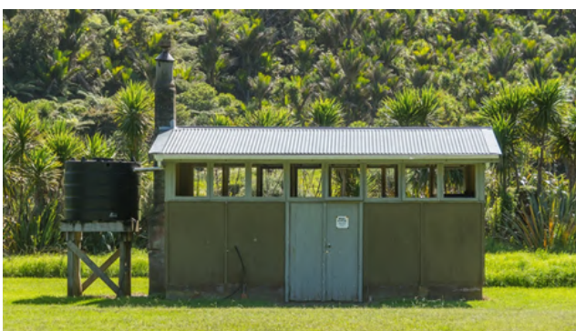
Figure 43. Nigel Hanlon Memorial Hut, Piha, North Elevation (Courtesy of Stefan Marks, 2024).
