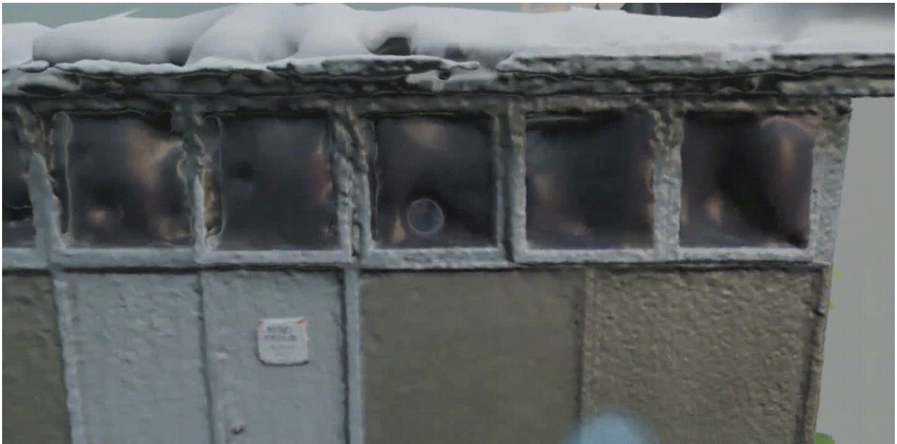
Figure 21. Smoothing of surfaces of the Nigel Hanlon Memorial Hut, Piha in Shapelab VR application, created by the Author.
