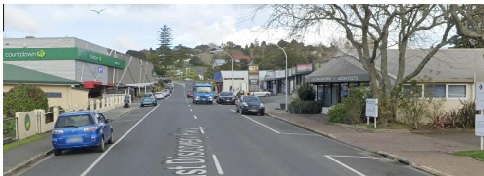
Figure 4.88: Twin Coast Discovery HWY in the Warkworth suburb in Auckland (Google Street View).
