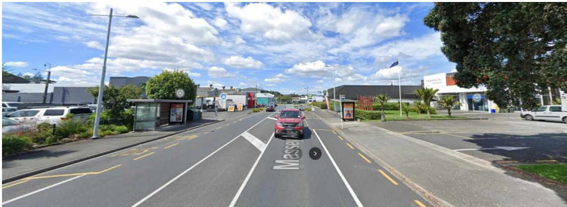
Figure 4.6: Massey Street in the Pukekohe suburb in Auckland (Google Street View).
