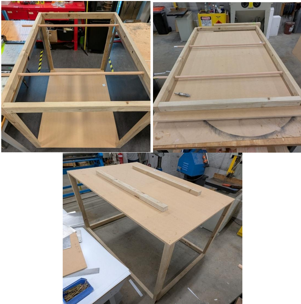
Figure 6.7-77 Wooden frame Work in Progress
