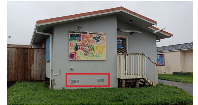
2. Floodwater could enter the building through the bottom vents.
