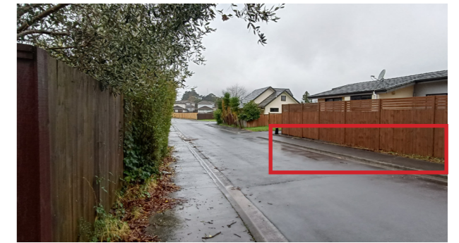
4. The bottom of the fences is enclosed, which will amplify runoff and prevent rainwater from passing freely.
