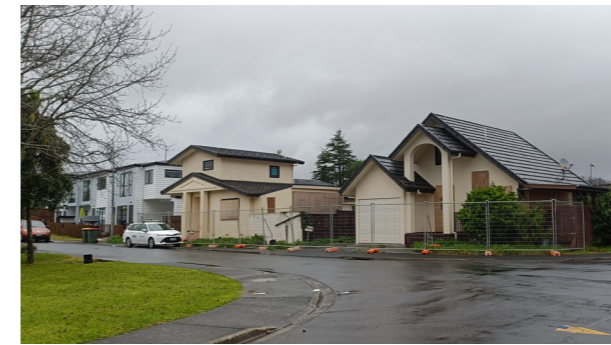
3. These houses were severely damaged by the flood, so they were bought out by the council.
