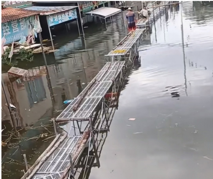
Figure 7.16 The construction process of the bridge (Huang & Huang, 2025)
