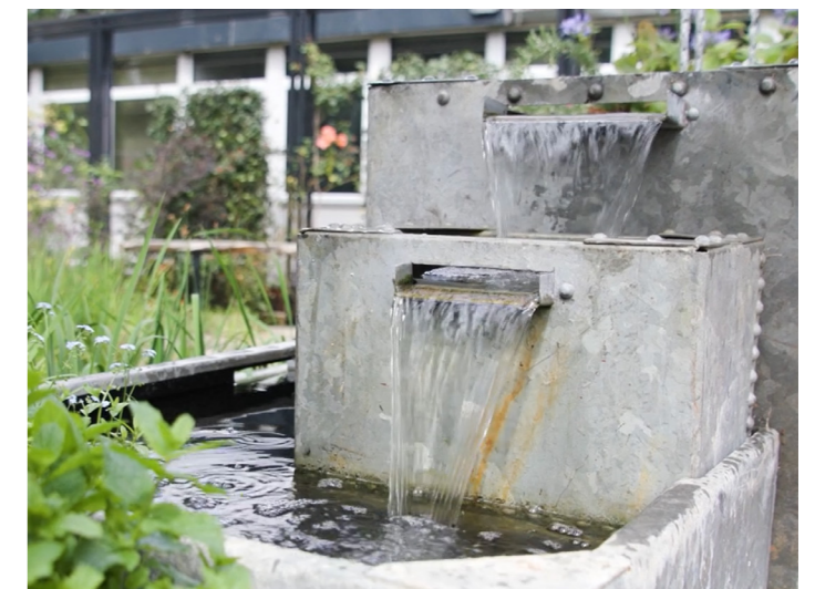
Below: Figure 7.24 Rain chains & Smart Rainwater tank
