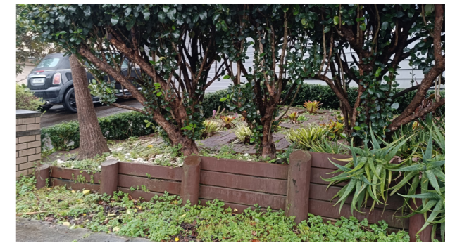
10. Retaining wall. This house located in a higher elevation area, was not listed as damaged after the flood.
