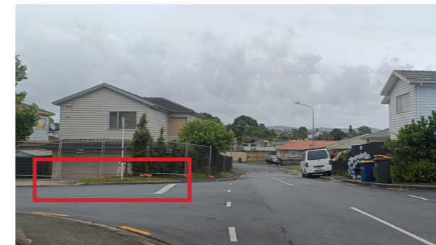
11. The ground level of this house is lower than the street surface.
