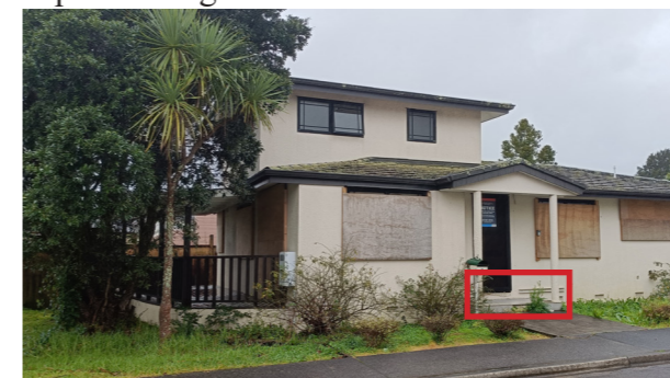
7. Elevation of door is not high enough.
