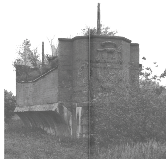
Figure 171: Bridge Fragment of Lange Brücke (The long bridge) at Forst (Studio Tom Emerson, 2012, p55)
