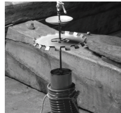
Figure 29: Climatized air duct heads within the ship (Hocker, 2010, p6)
