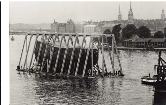
Figure 27: Structure for Temporary Museum, the Pontoon with the Concrete Beams Leaving the Dry Dock (Håfors, 2010, p23)
