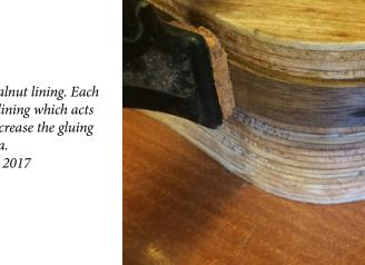
Figure 141. Detail of the walnut lining. Each side has a front and back lining which acts to provide stability and increase the gluing surface area. Author's image 2017
