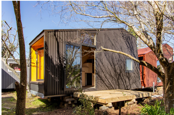
Figure 10. Whare Tahī Exterior, 2021 . SGA Ltd for Vision West Waka Whakakitenga. Photograph Ross Keane - SGA Ltd.
