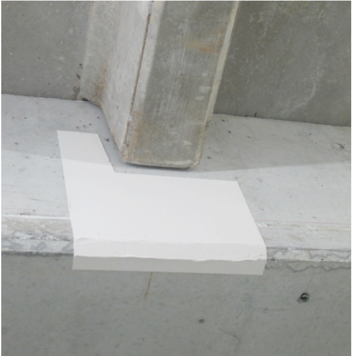
Subject[ed] Matter , Installation detail, Gib Stopping Plaster (applied Directly to concrete wall), AUT, 2013
