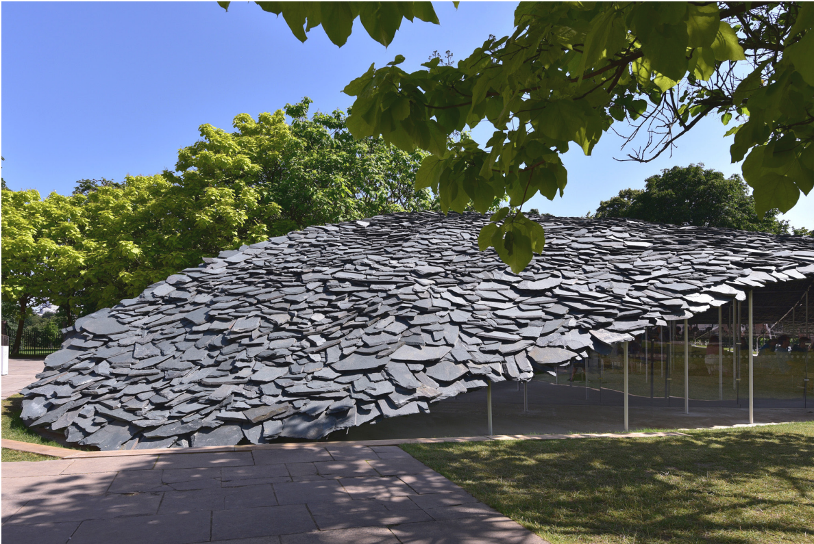
Figure 48. Junya Isigami. Serpentine Pavilion 2019. Architectural installation. Serpentine Gallery, London. Designed by Junya Isigami + Associates. Photography © 2019 Iwan Baan. [Replaced with Serpentine Pavilion - 2019, Images George Rex, CC BY-SA 4.0 < https://creativecommons.org/licenses/by-sa/4.0/ >, via Wikimedia Commons.]
