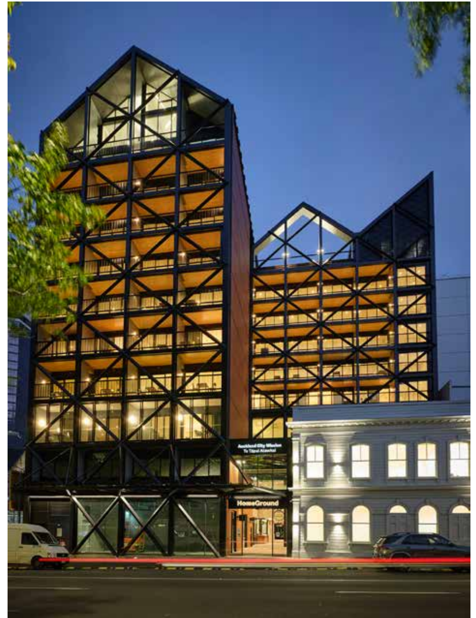
Figure 8 Homeground (Stevens Lawsons Architects, n.d.)
