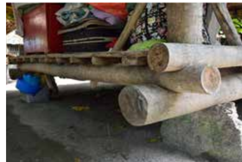
Figure 55 Base structure of a traditional hut (Travel tour Guide, 2015)
