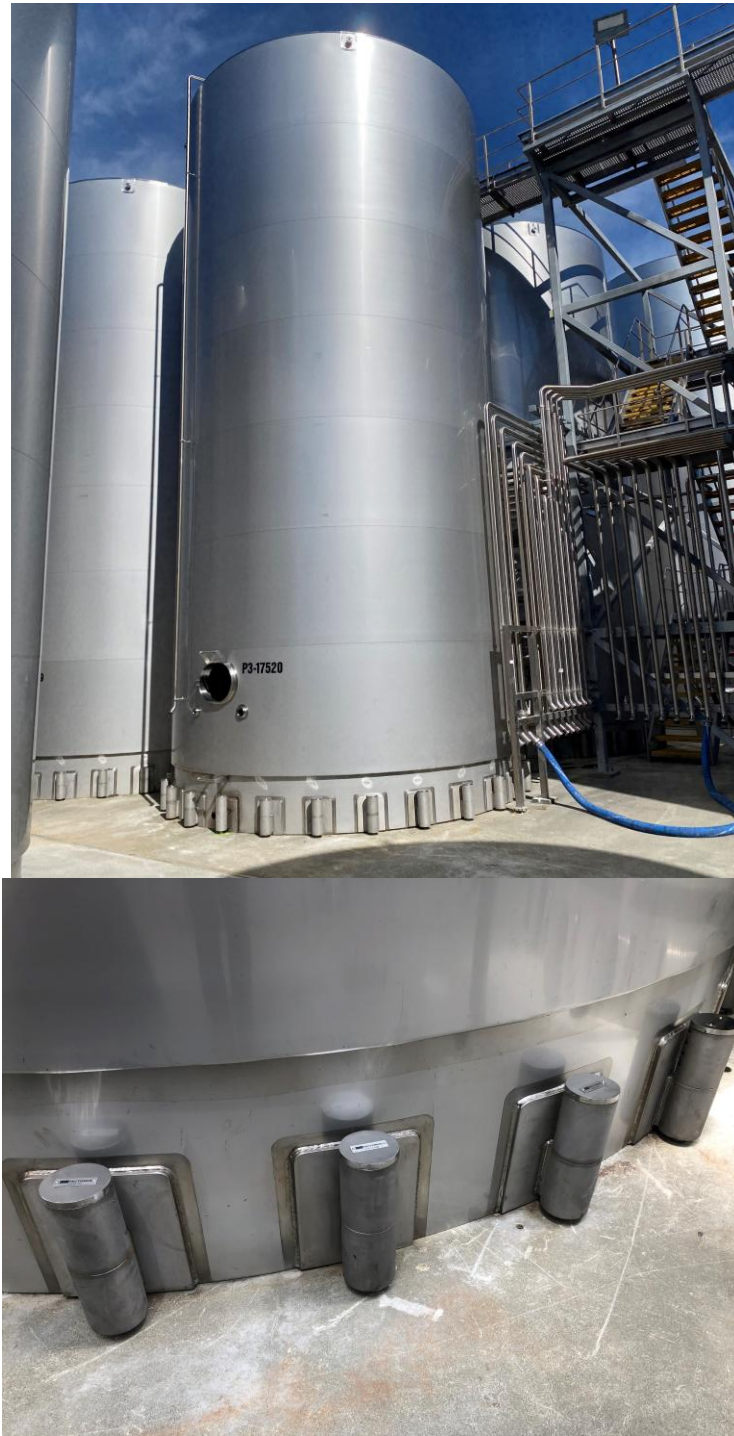
Figure 6-16: Implemented RSFD as anchorage system for wine tanks
