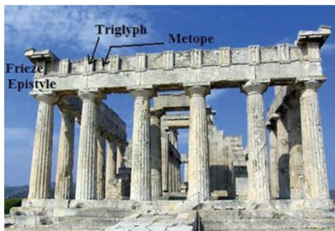
Figure 2-1: View of a temple of Aphaia, Greece. Free-standing columns, standing for more than 2500 years (Makris and Vassiliou 2014)
