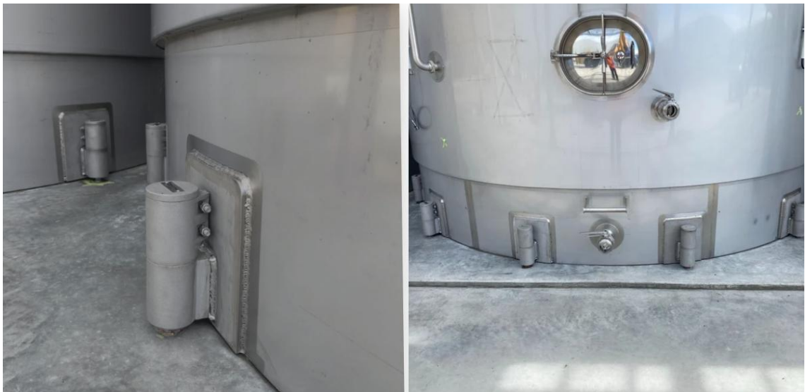
Figure 6-18: Implemented RSFD as anchorage system for wine tanks
