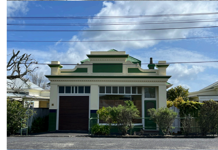
26 Queen Street, former shop
