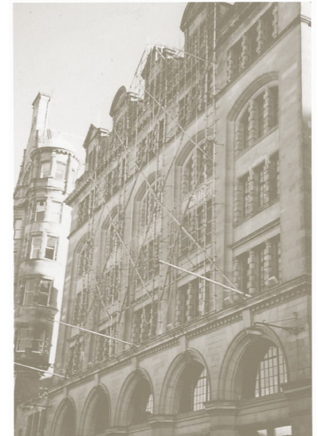
Figure A.03: "Bamboo scaffolding outside the exhibition hall at the 'Hong Kong Tomorrow' exhibition in 1996, at Edinburgh in Scotland. The scaffolding was erected by master scaffolder Choi Keung, instructor at the Construction Industry Training" (sourced from Waters, 1998)
