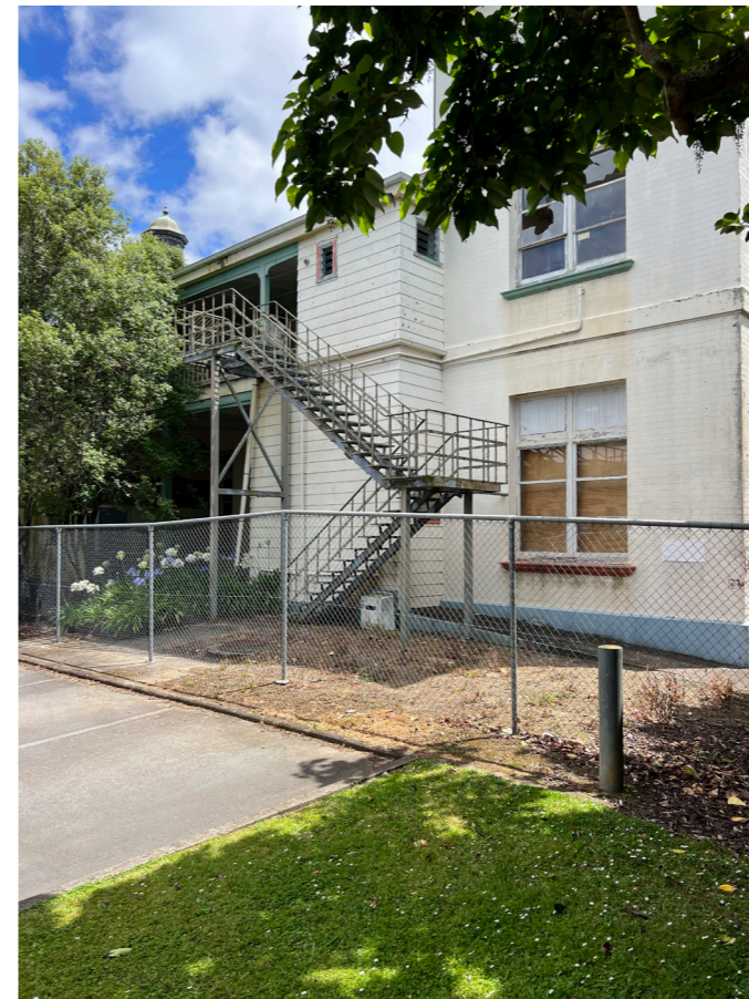
Figure 15 View of the northeast fire egress addition and partially walled-in verandas. A similar stair was removed from the Eastern Wing.
