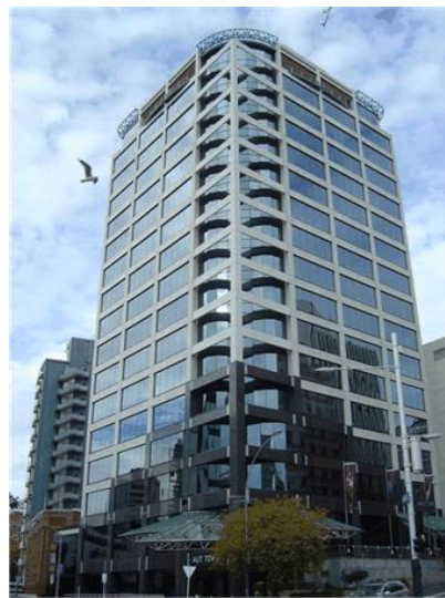
Figure 12. External view of WT tower building.
