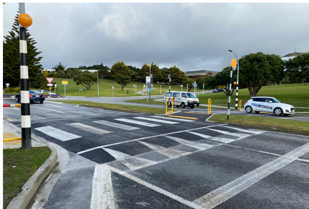
Figure 152 - Pedestrian priority crossing installation across 4-lane road in Porirua. From Titahi Bay Road pedestrian crossing by Waka Kotahi, 2022 ( https://www.nzta.govt.nz/safety/partners/road-safety-resources/safe-system-case-studies/titahi-bay-road-pedestrian-crossing/ ).
