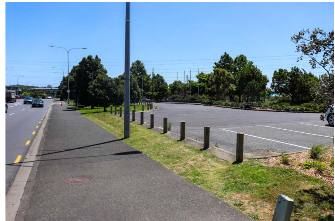
Figure 149 - Playground Carpark, Olympic Park - Photograph by Author
