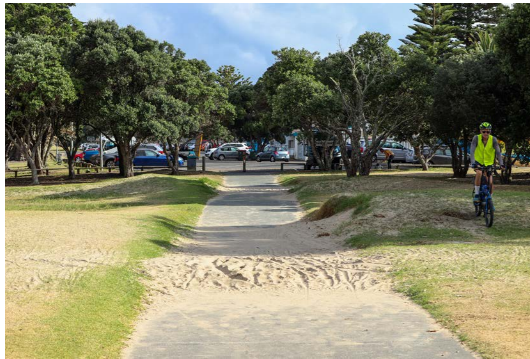
Figure 49 - The sandy lifestyle doesn't come with out it's downsides, Orewa Beach - Photograph by Author
