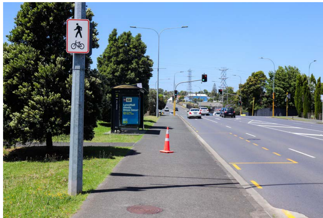
Figure 147 - In lane bus bay and Bus Stop, Olympic Park - Photograph by Author
