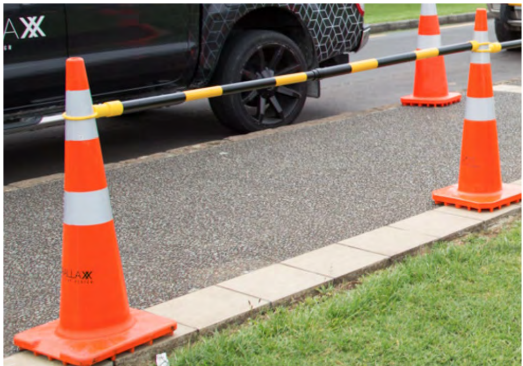
Figure 34 - Cone Bar use for access prevention (New Zealand)
