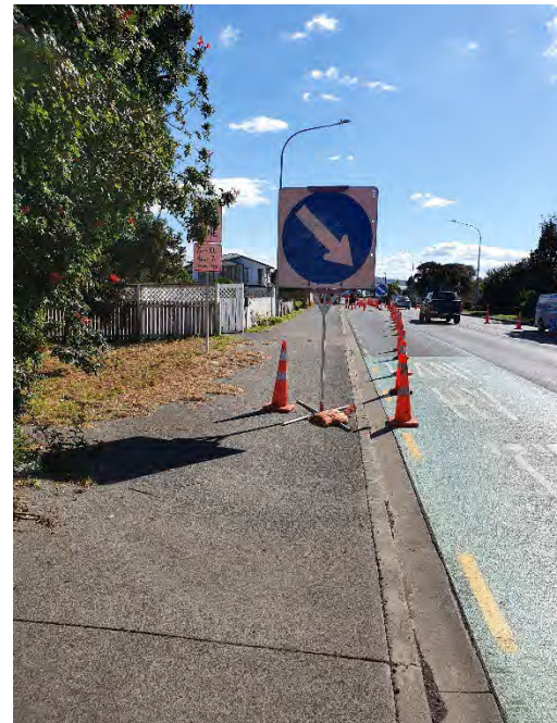
Figure 47 - TTM sign impacting VRUs 2
