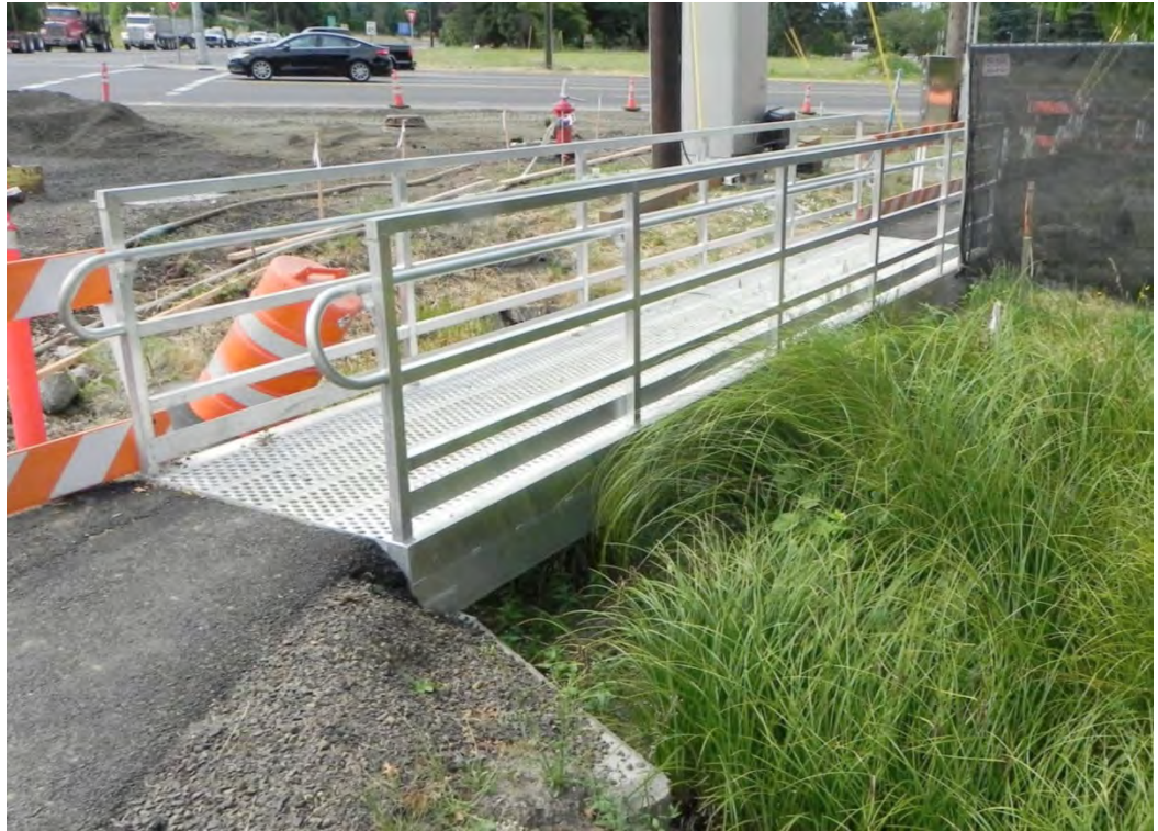
Figure 42 - Temporary walkway bridge example(ODOT, 2018)
