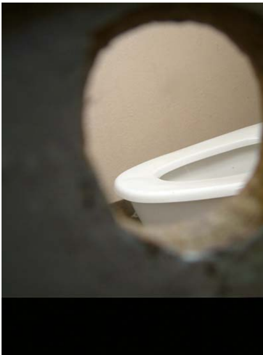
Hand drilled hole – public toilet Auckland
