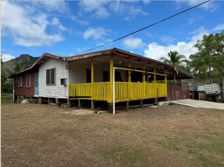
Figure 4.1.5. My (maternal) grandfather's house located in Buleleka, Labasa (photo by the author).
