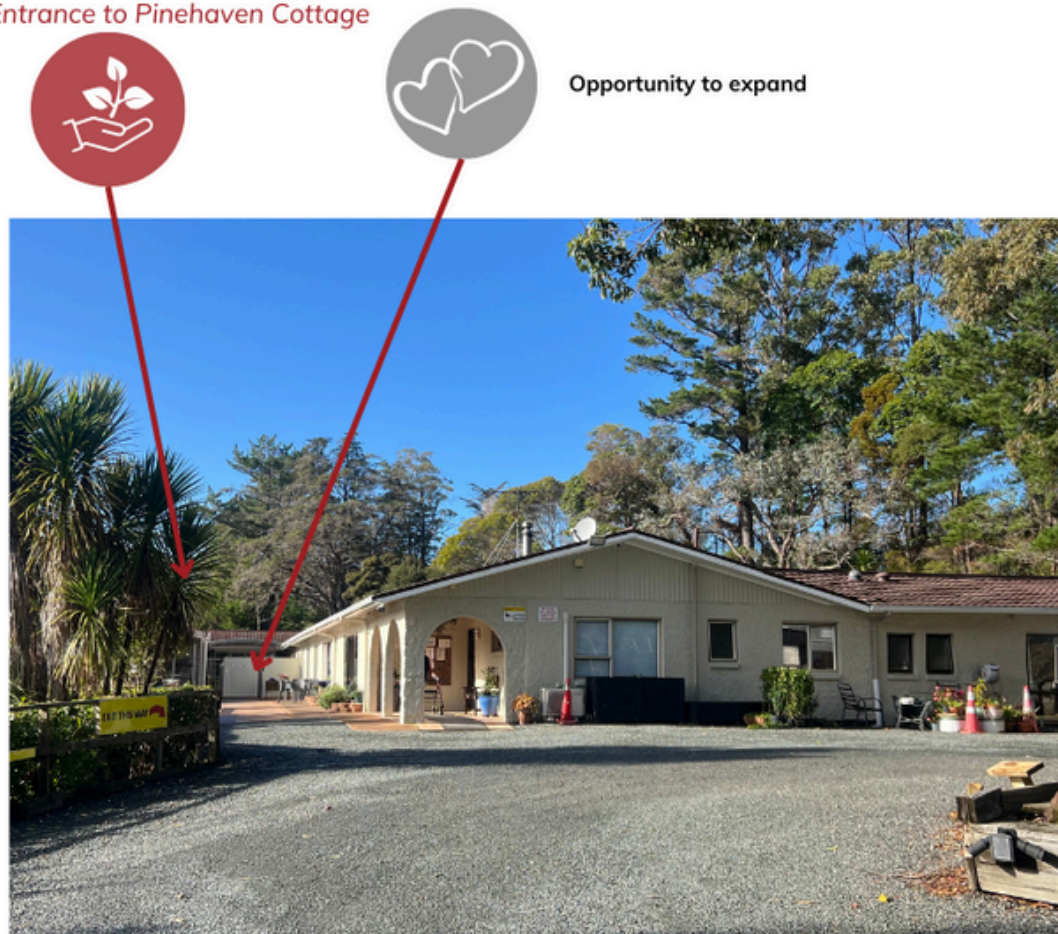
Figure 53 Exterior of Pinehaven Cottage
