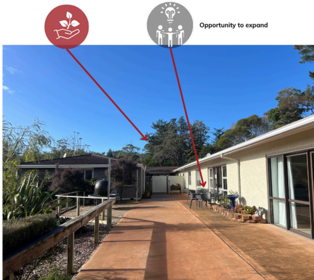
Figure 50 Entrance to Pinehaven Cottage
