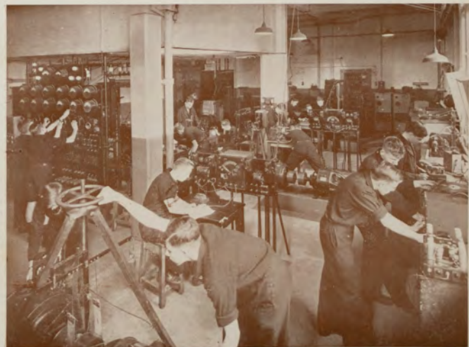
GENERAL VIEW, ELECTRICAL MACHINE LABORATORY
