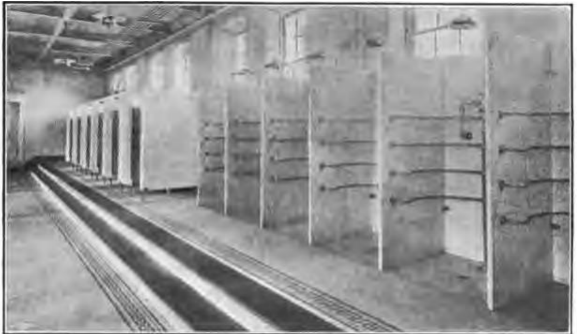
FIG. 60. VIEW OF SHOWER BATHS FOR EMPLOYEES IN WESTERN ELECTRIC MACHINE WORKS, NEWARK, N.J.
