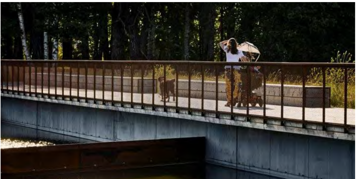
Figure 22: The Stormwater Pond at Exercisfältet, White Arkitekter, 2021
