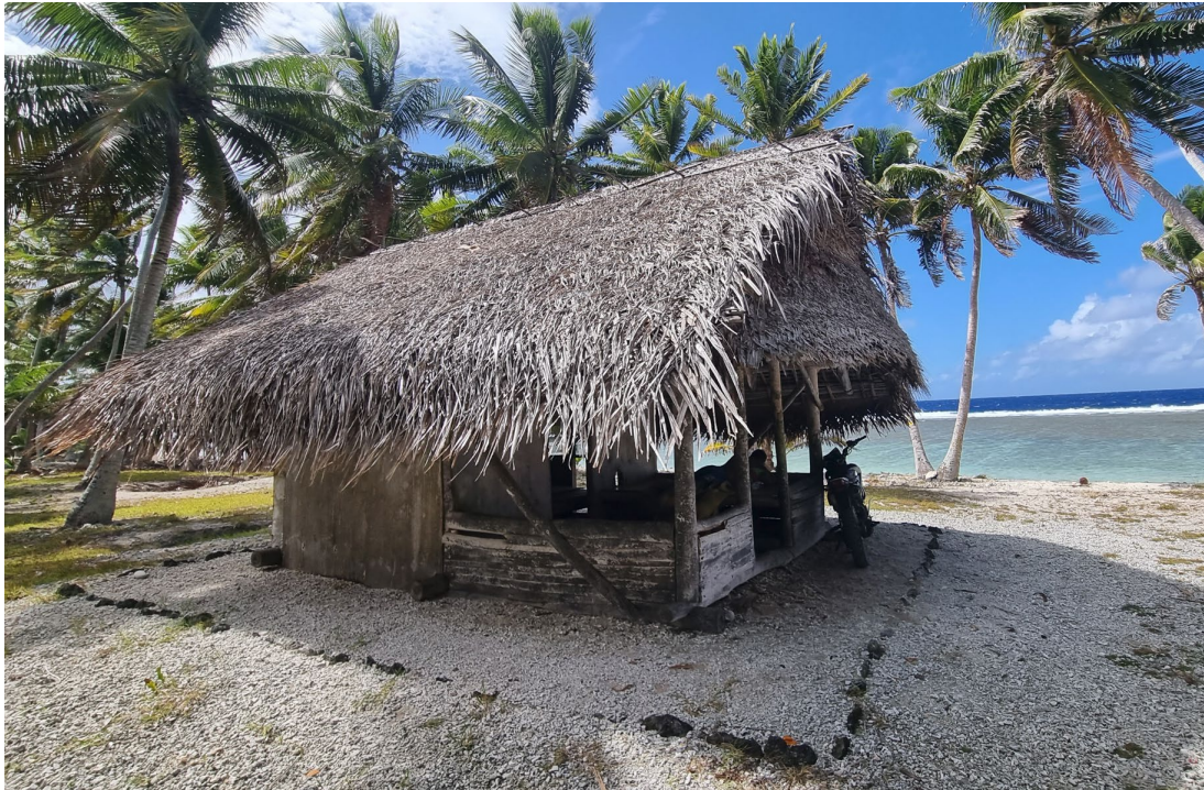
Figure 32: Platform stones raised around building. Note 'yoka' bracing
