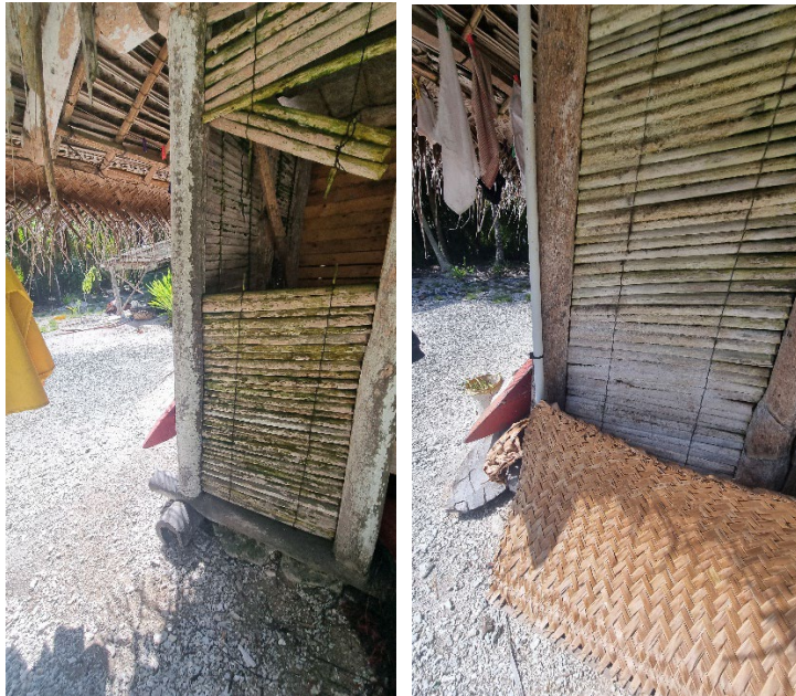
Figure 30: Timber wall slats, & takapau on ground
