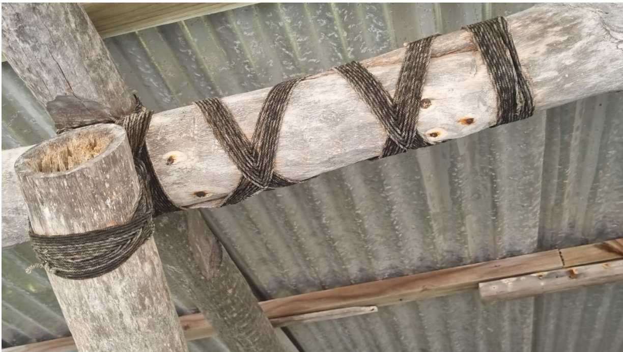
Figure 23: Yimu Wakawiwi or Paiokiole lashing technique, old meeting house Nassau, 1987
