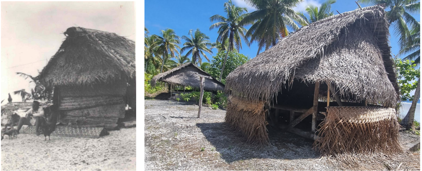
Figure 28: Wall mats, pola & takapau . Note ;yoka bracing
