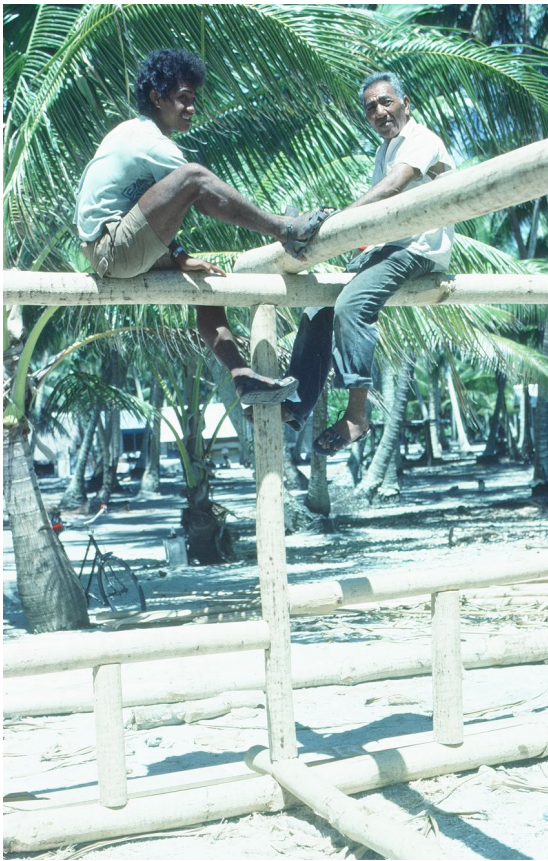
Figure 41: Wale atua house with tie beams notched into top wall plates
