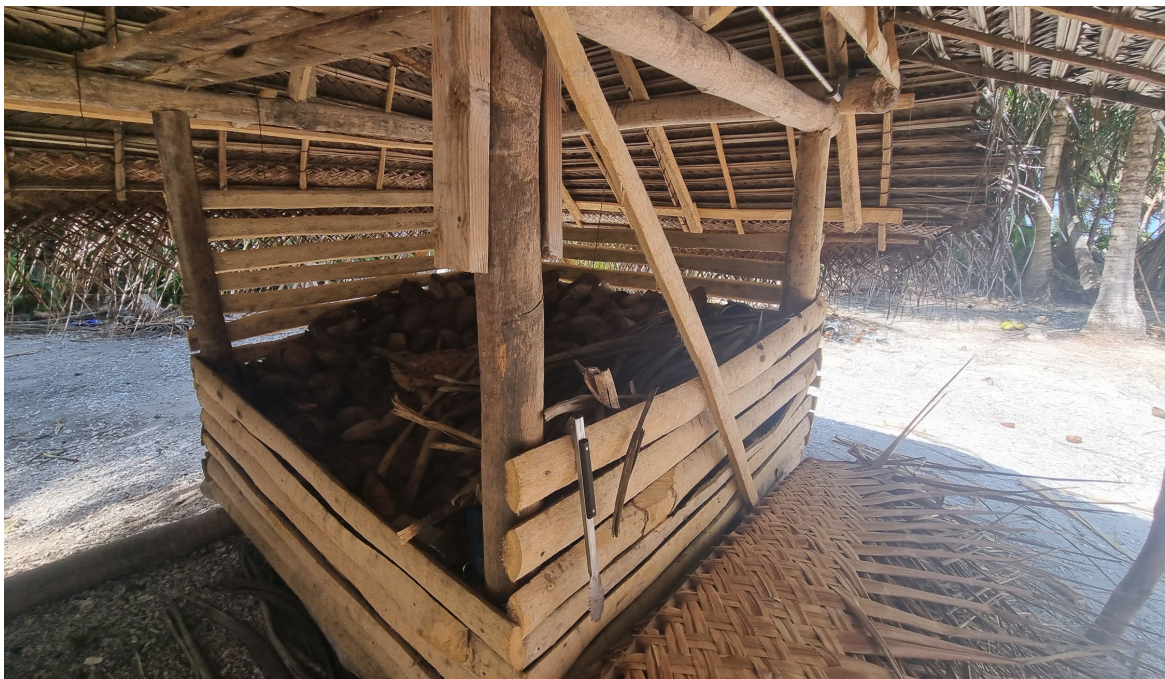
Figure 37: Small store house, interior view. Note 'yoka' bracing elements
