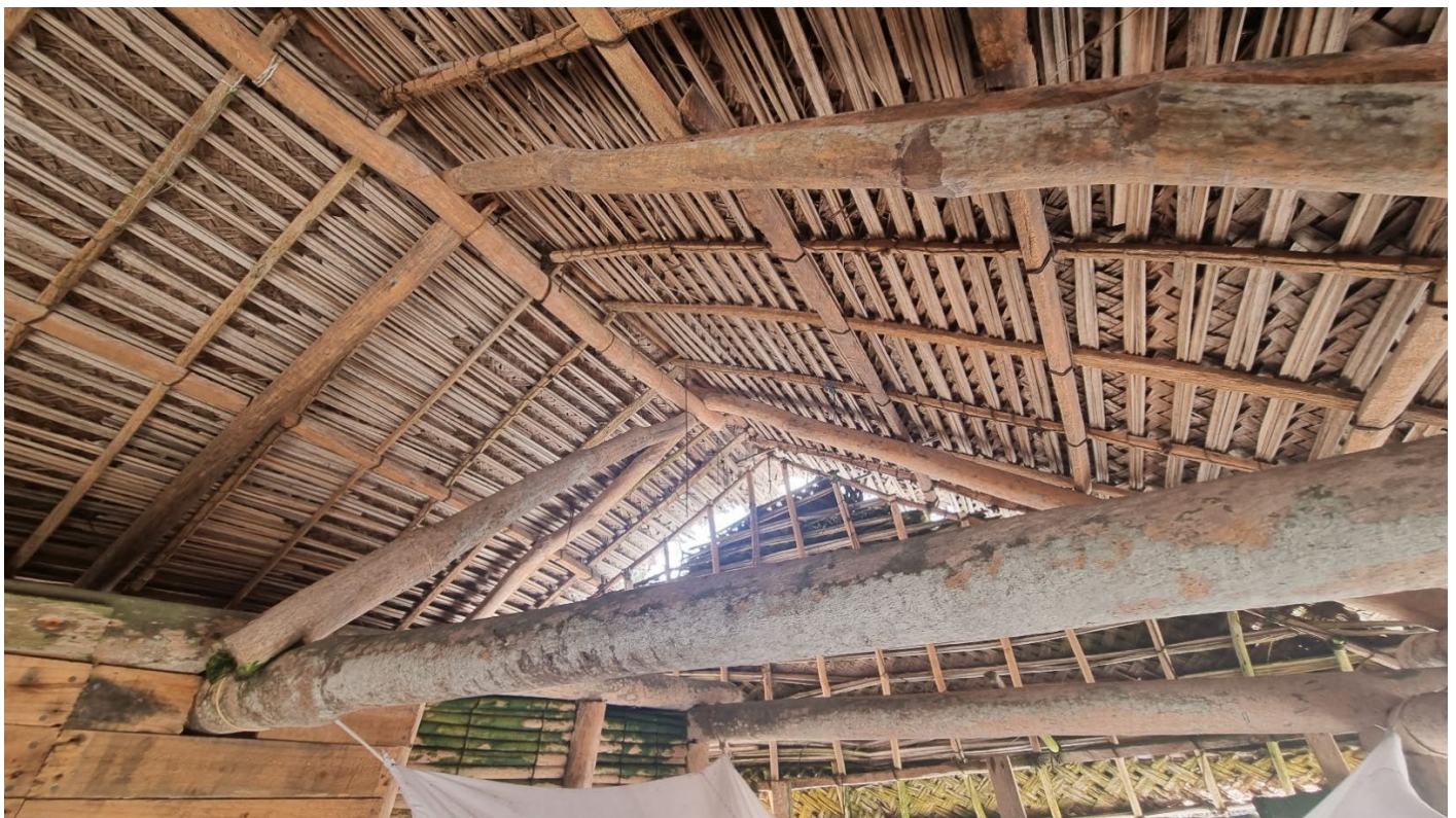
Figure 13 Underside of 'wale wakayamoa style, note diagonal 'oka' roof bracing
