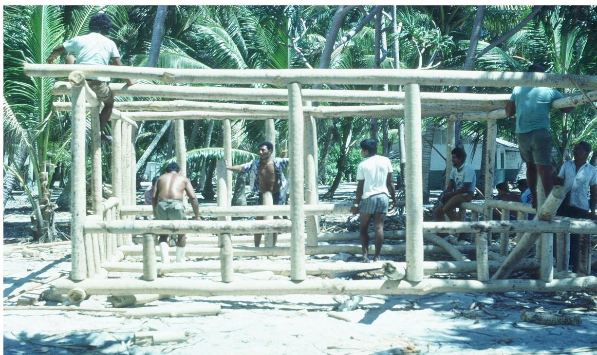
Figure 40: Wale house under construction
