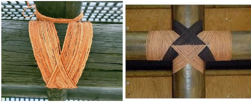
Figure 54: Tongan examples of kafa lashing techniques
