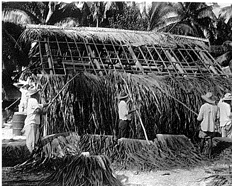
Figure 25: Thatching new roof with lau wala
