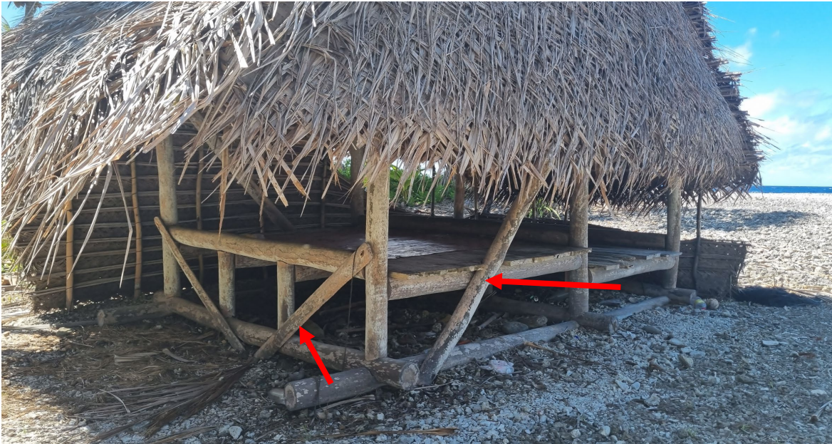
Figure 34: Typical wakayamoa type, sleeping house (wale). Note 'yoka bracing
