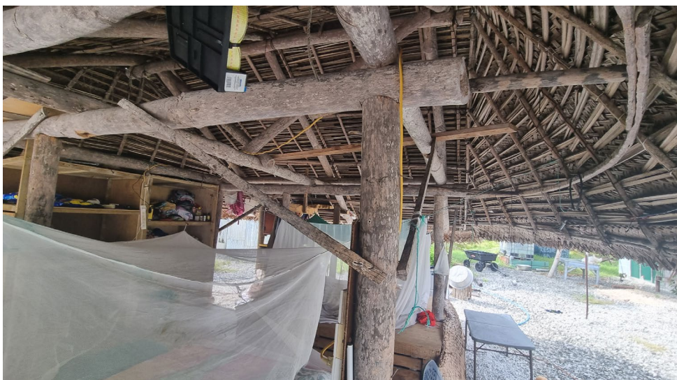
Figure 26: Gable end eaves, showing oka (tiebeams) kayo (thatch rafters) and talava (purlins)
