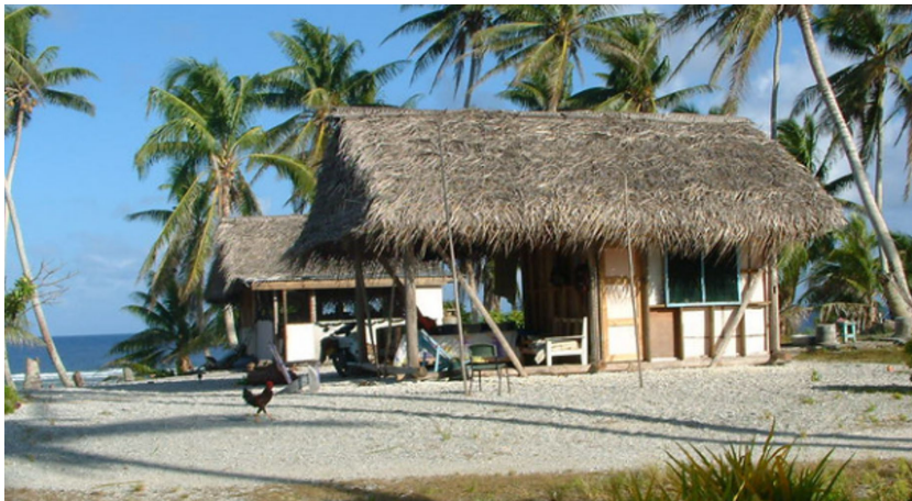
Figure 508: Modern traditional wale house with 'yoka' bracing
