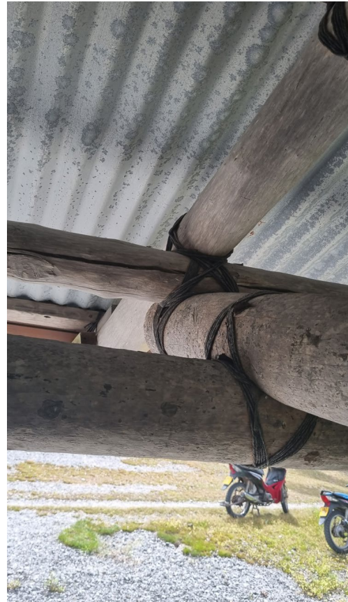
Figure 41: Wale atua house with tie beams notched into top wall plates
