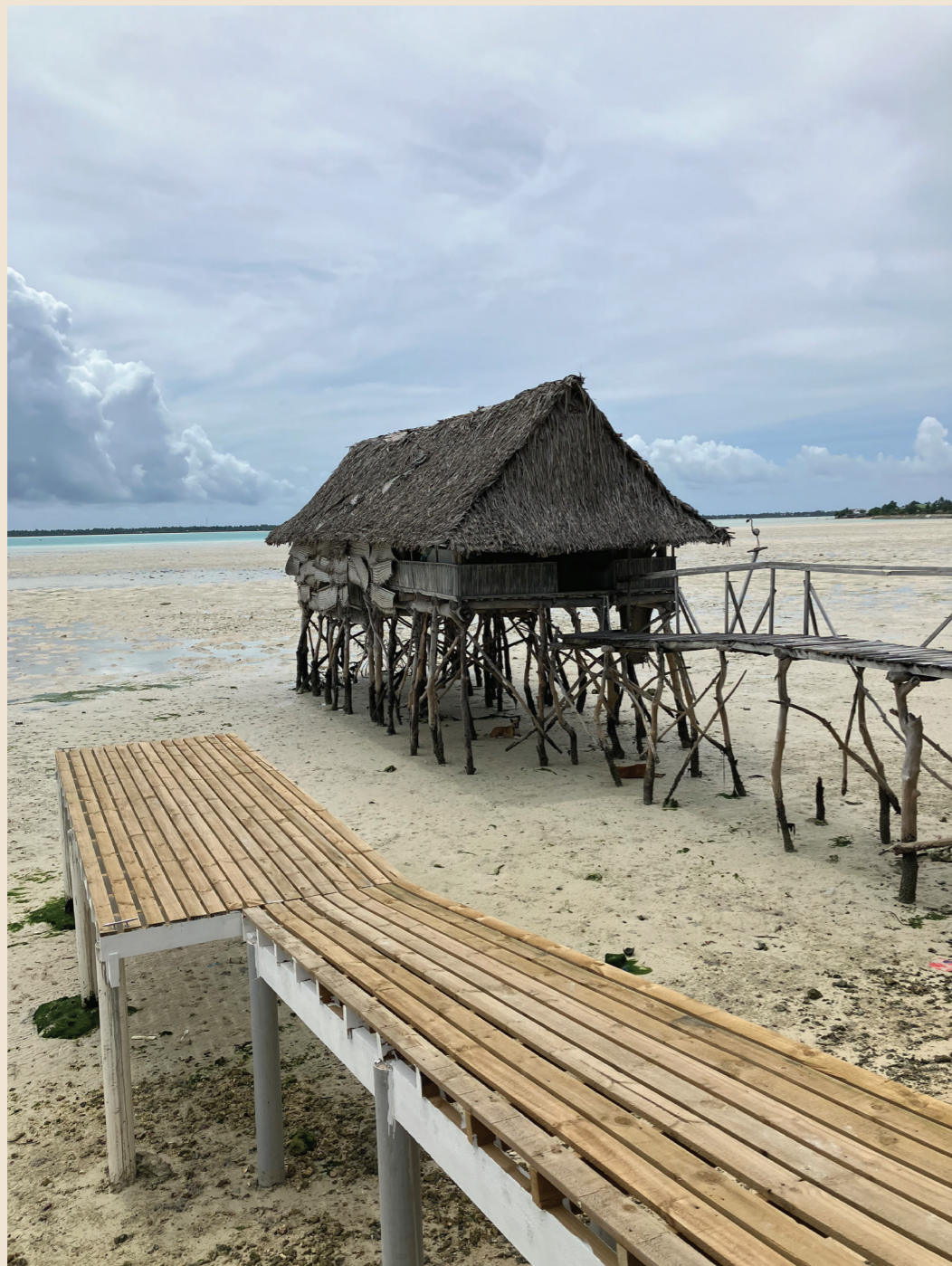
Figure 32. Image: New & old wharf structure in Kiribati
