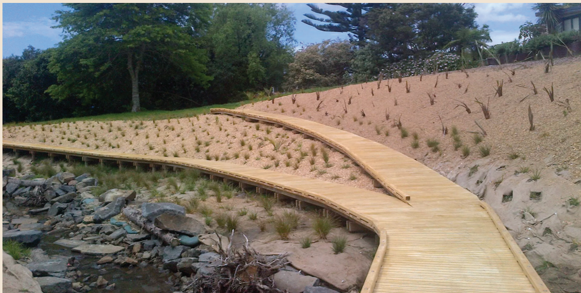
Figure 31 . Image: The Auckland Council Stormwater Project
