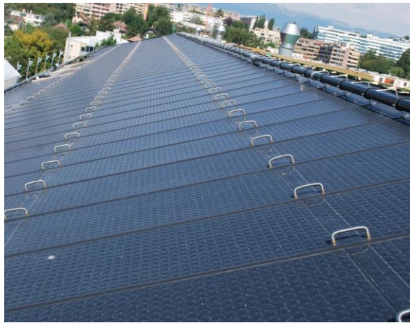
a. Unglazed stainless steel flat plate collectors
