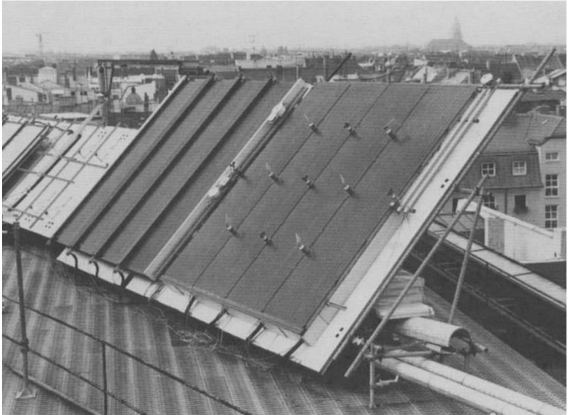
Figure 7: Outdoor set up of roof mounted Solar thermal collector (Soltau,1992)
