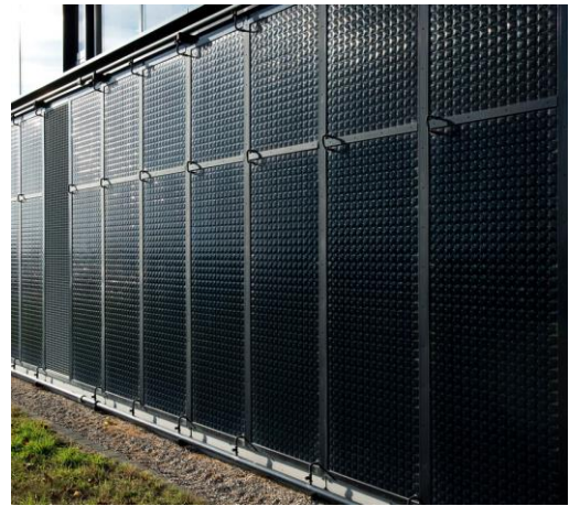
b. Façade cladding of unglazed collector
