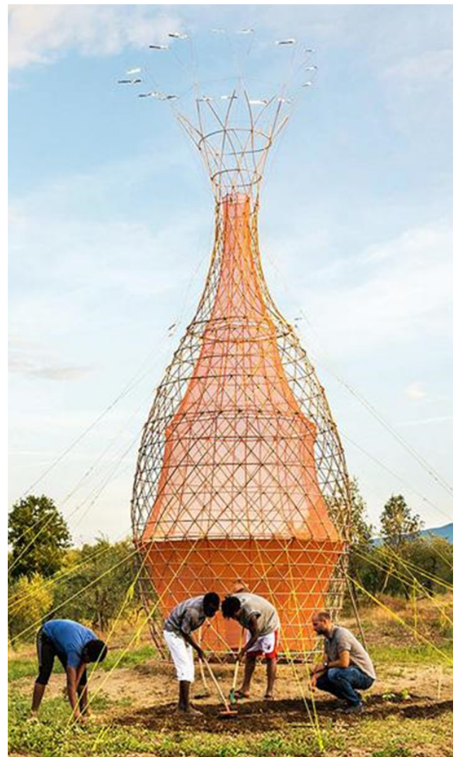
Figure 27. © Warka Water. Bamboo structures positioned to collect and harvest rainwater, photograph, 2015.
