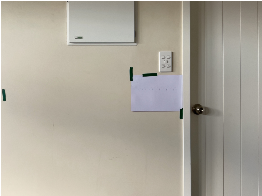
Figure 3.15: Each increment on the paper placed on the wall is an increment of 50mm.
