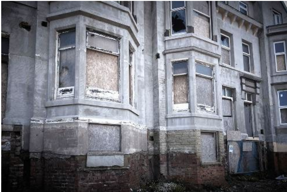
Figure 2. Abandoned hotels on the front of Blackpool promenade. Photography by David Sinfield. July 2023
