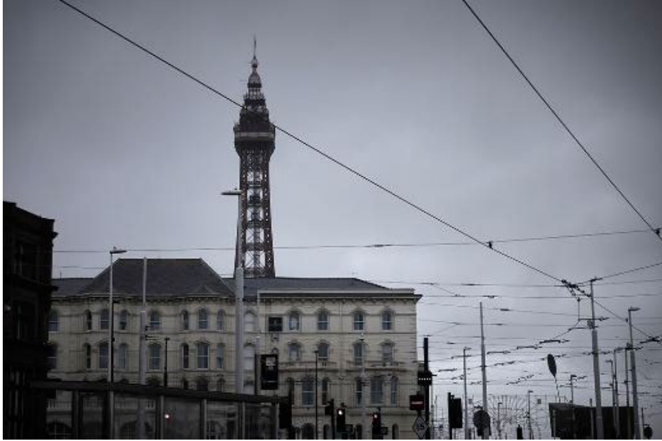
Figure 4. Blackpool Tower and Tramway electrical cables. Photography by David Sinfield. July 2023
