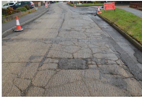
Figure 2.4: Block Crack [2]
