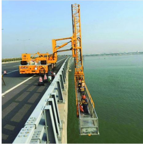
Figure 2.6: Example of manual crack inspection on a bridge [3].
