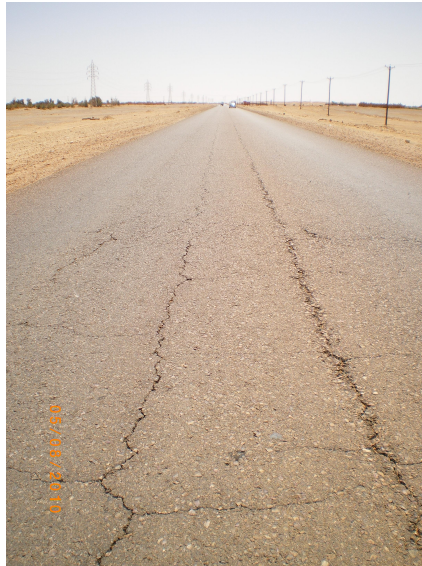
Figure 2.1: Longitudinal Crack [2]
