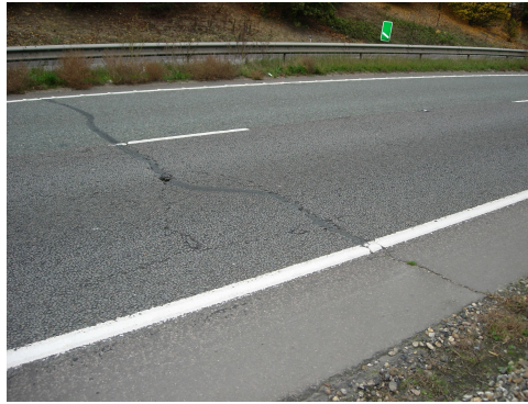
Figure 2.2: Transverse Crack [2]
