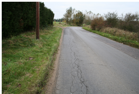
Figure 2.5: Edge Crack [2]
