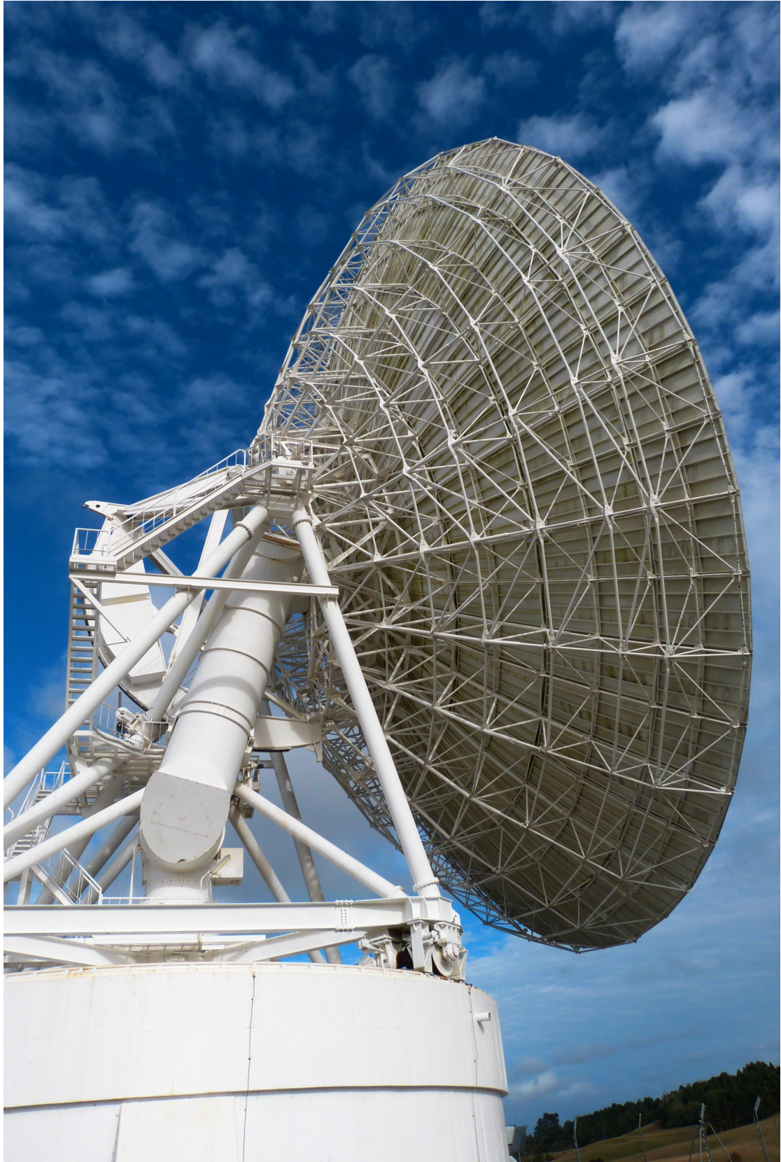
I worked with the team from the Institute of Radio Astronomy and Space Research, AUT University between 2010 and 2014 converting this former satellite communications 30m dish of Telecom NZ to a Radio Telescope Woodburn et al. (2015) . Credit: Stuart Weston
