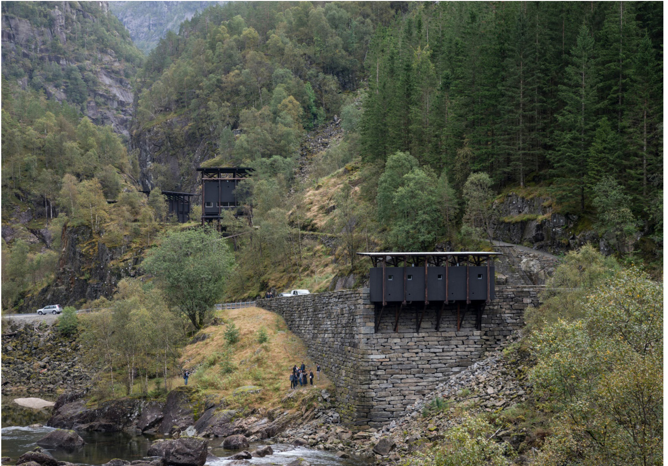
Figure 47. Peter Zumthor, Allmannajuvet Zinc Mine Museum, 2016, three of the four buildings placed along the walking track with the incentives of finding the next building from the atmospheric experience
